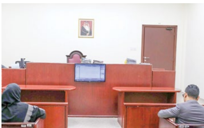
An LCD screen installed at a courtroom.
